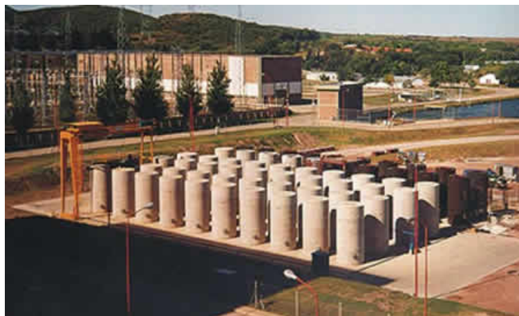
Figure 2. Argentine storage of SNF placed inside concrete silos (www.invap.net)
