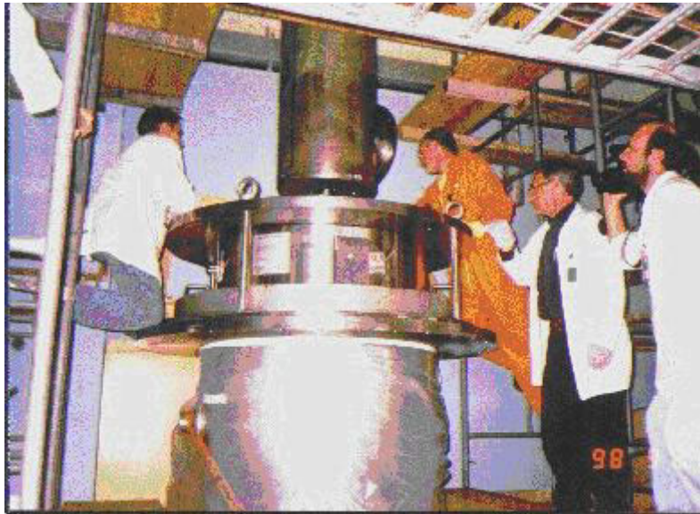
FIG. 1. View of the transfer cask used to transfer the assemblies to the transport cask.
